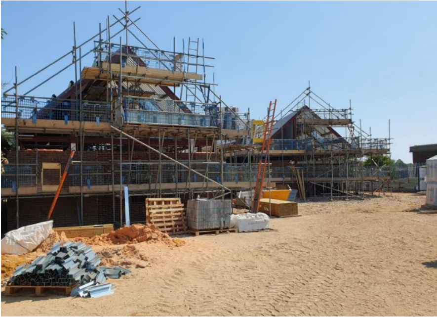
Photo of construction of the new Keystone Centre.
