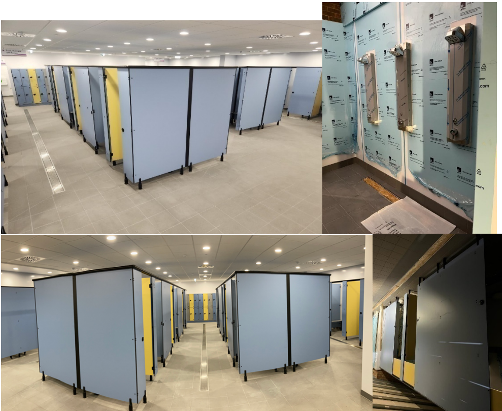
Photo of refurbished wet change at Arun Leisure Centre
